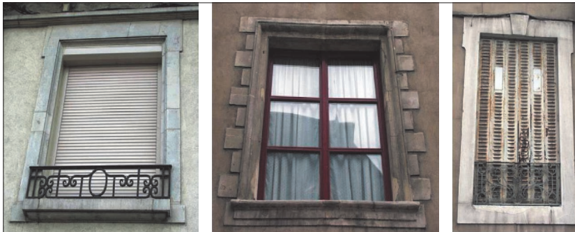
Pictures of openings in Nancy and Montreal
