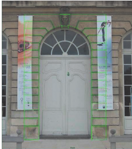
► Figure 8. Adjustment of the parameters of the door with the help of a picture.
